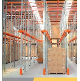
Drive-In & Drive-Through Racks offer the ability to store a large number of similar loads in a smaller area. Selectivity is sacrificed, but storage density is outstanding. Drive-in Racking can store up to 75% more pellets in the same space than selective rocking depending on your application.
